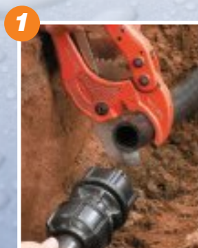
1 Cut the pipe square. There is no need to chamfer or lubricate the pipe.
