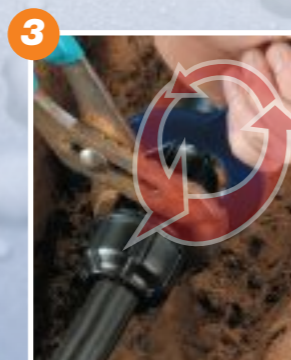
3 Tighten the nut by hand, and then with a wrench to the point where the nut is touching the flange on the body of the fitting. Do not tighten beyond this point.
